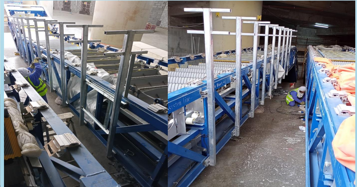
LUSAIL PLAZA TOWER: Escalator Framing Support System
